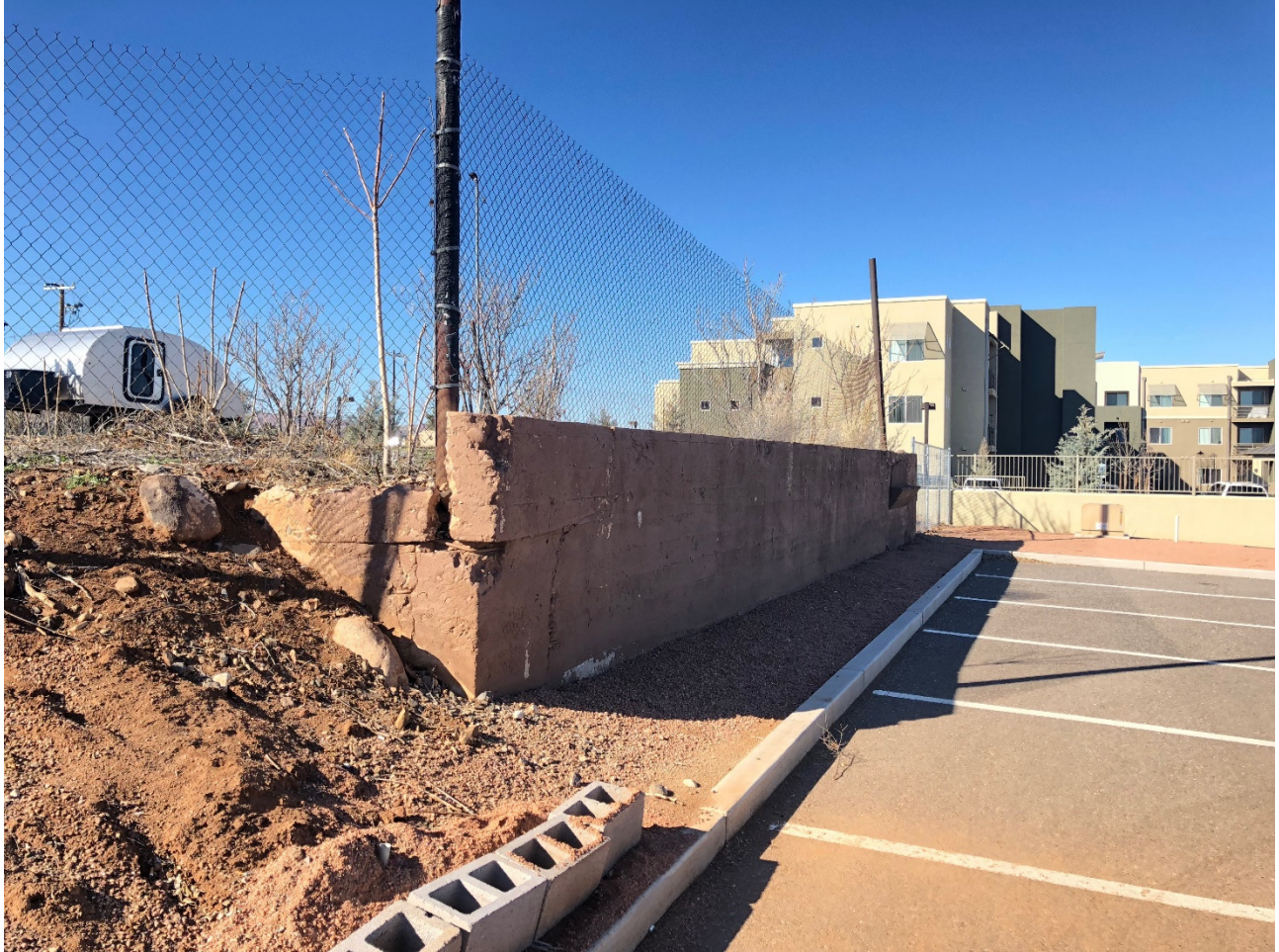
Figure 2. Existing Retaining Wall
