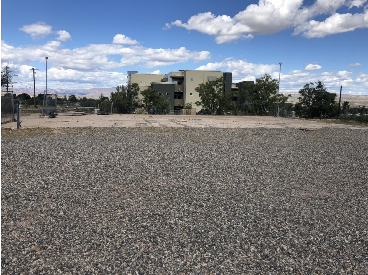
Figure 5. Existing Concrete Pad
